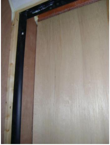
Install 1/8 panel with grain running vertically so it can flex into the cavity. Panel should be approximately 23" x 38".
