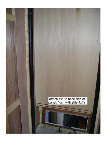
Attach a 1x1 on the lower back side of the panel flush with the side blocks. This is for attaching the lower cover plate.
