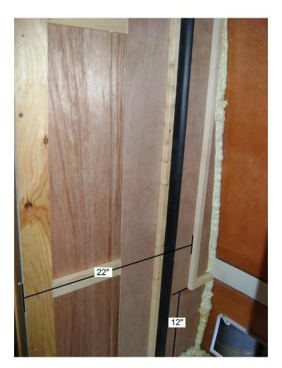
Mark 12" up from the fridge deck and 22" back from the front edge of the cabinet. Attach a 1x1 across the bottom (approx. 4.5") and one from the top of the bottom block up (approx. 36")
