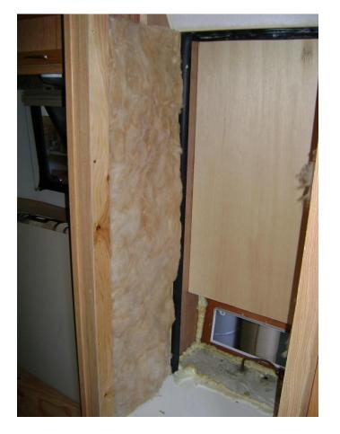
Install approx. 1.5" thick insulation on the sides
