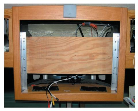
I chose 1 1/2 aluminum angle, mounted to the sides with 3/4 inch plywood attached to the back of the angle. The back of the angle was placed at the dimension of my depth (2 11/16"). Not showing is a 2 x 2 that is screwed and glued horizontally across the back of the plywood for stiffness.
